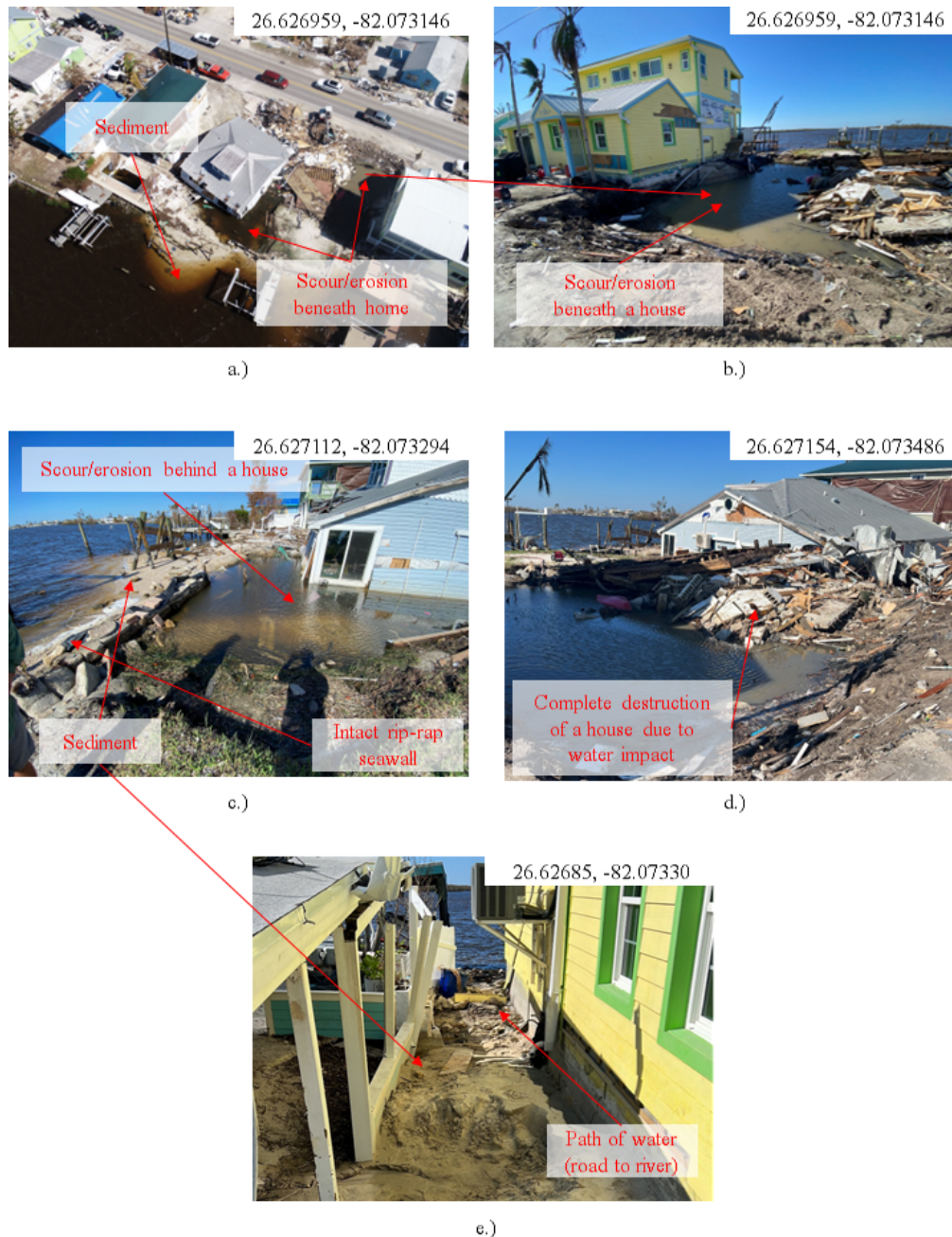
Figure 4.10: Severe damage and erosion to houses on Matlacha Isle, located on the left side of Pine Island Road: a.) drone image showing sediment accumulation, indicating the direction of high water flow with evidence of scouring and erosion beneath the foundation of two homes; b.) ground image depicting evidence of scouring and erosion beneath the foundation of the yellow house; c.) ground image of the back of the blue house reveals transportation of sediment, indicating the direction of water flow from behind the intact rip rap seawalls. The settlement of the house is also visible due to erosion and scouring beneath its foundation; d.) One house has been completely destroyed, with debris and water accumulation observed at the site; e.) accumulation of sediment suggesting water flow direction from Pine Island Road to the back of the houses, which is opposite to the predicted path.
