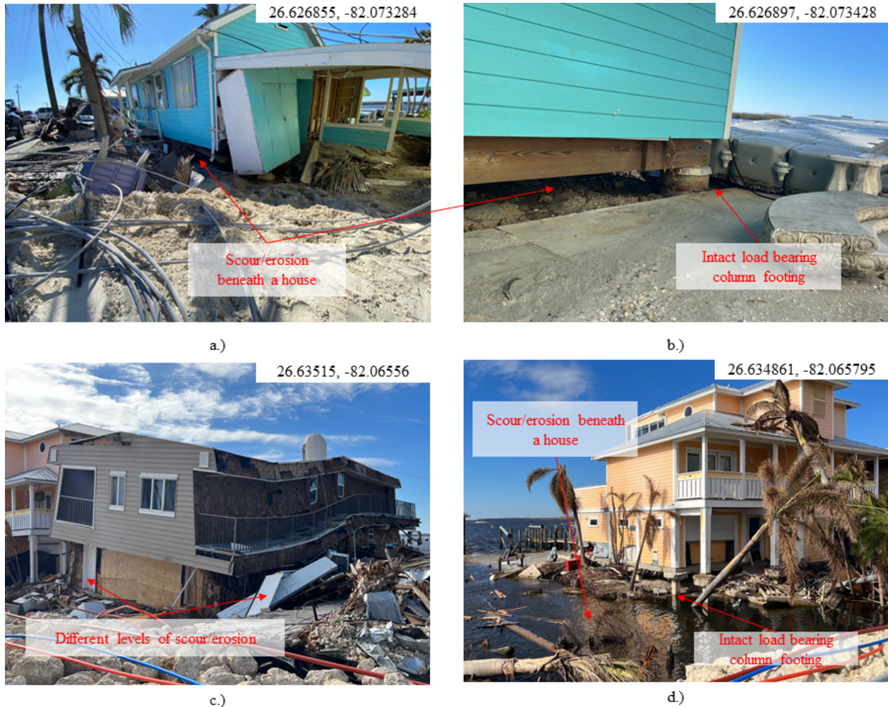
Figure 4.8: East entrance to Matlacha: a.) accumulation of sediment and debris and erosion and scour underneath the house; b.) load-bearing column without any damage to the footing during the scour and erosion process underneath the foundation at the back of the house; c.) different levels of erosion underneath the house's foundation resulting in a differential settlement; d.) the load-bearing columns remaining intact without any damage, despite a significant amount of scouring and erosion
