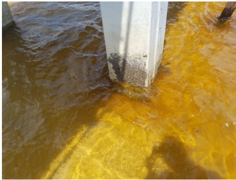
Figure 2.15: Scour at the base of the Ft. Myers beach finishing pier. Coordinates: 26.449636, - 81.944446 (Stark & Hudyma, 2017)
