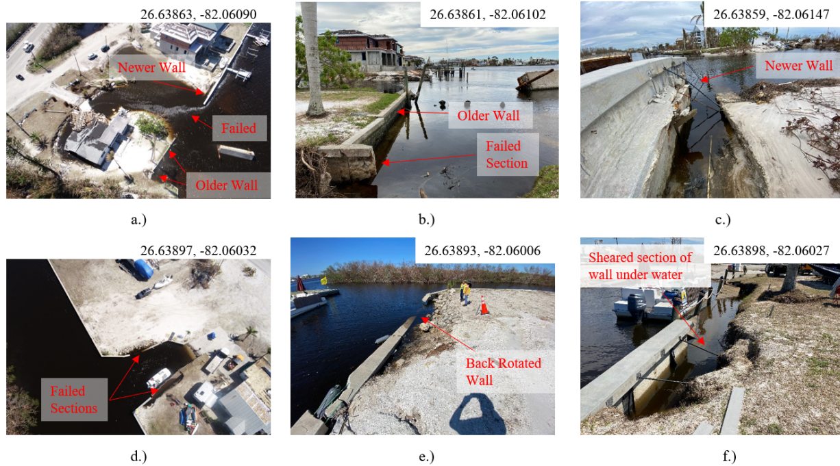
Figure 4.4: Damage to retaining walls near the intersection of Shoreview Drive and Pine Island Road in Matlacha Isles-Matlacha Shores: a.) drone image showing failed section of retaining wall believed to have occurred at the interface of older and newer section of the seawall; b.) older portion of sea wall; c.) newer section of sea wall; d.) drone image of failed retaining walls at a boat ramp; e.) back-rotated sea wall on one side of boat ramp; f.) sheared portion of a seawall underwater on other side of the boat ramp.
