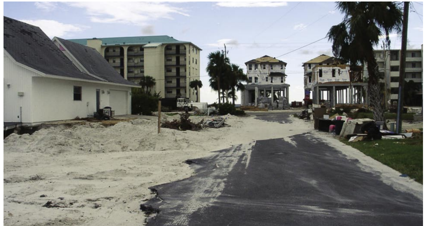
Figure 2.10: Scouring of the road and damage to the infrastructure in Fort Myers Beach. Coordinates: 26.45060, -81.95103
