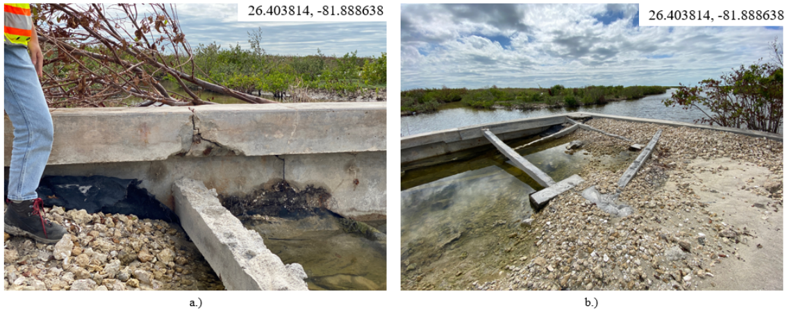
Figure 4.36: Southern end of the Fort Myers Beach: (a) ground photo depicting a broken anchor of a sea wall showing the tie-back used in the anchor system; (b) ground photo of the anchoring system showing cross beam tie backs and dead man weights
