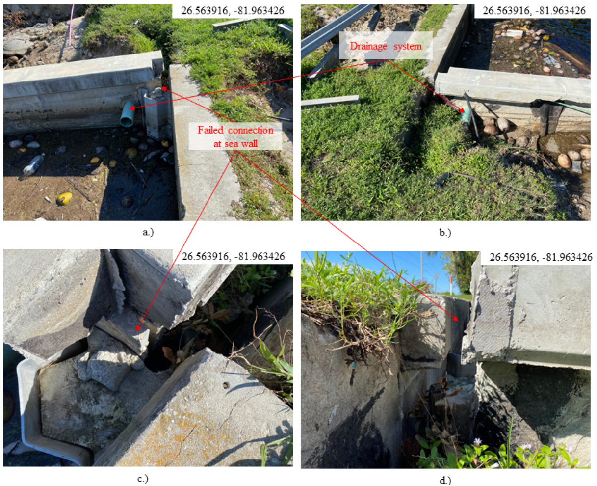
Figure 4.16: Ground photo of the erosion-induced sinkhole on the right side of the canal: (a) drainage pipe is visible and might have been the primary cause of the failure at this section (b) drainage pipe in the vicinity of the cavity created by erosion; (c) failure of the retaining wall as a result of the vacuum effect of the voids created in the soil; (d) back of the failed retaining wall showing the breakage and displacement
