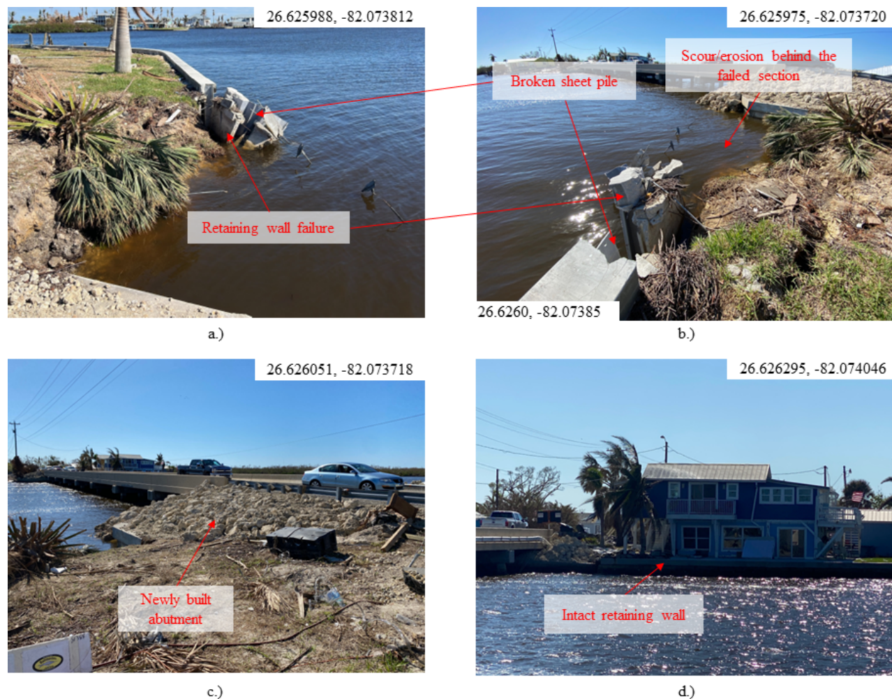
Figure 4.12: Ground photo of the upper side of the bridge: (a) remaining piece of the broken seawall showing breakage in the sheet pile's connection; (b) scour and erosion as a result of the failed seawall behind the failed section causing more damage to the wall and accelerating the deterioration; (c) ground photo of the newly built abutment for the bridge; (d) ground photo of the lower side of the bridge showing the intact seawalls that had no damage.
