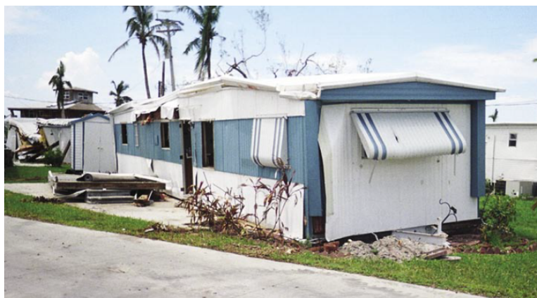
Figure 2.8: An older manufactured home that was uprooted off its base and damaged the building itself in Pine Island. Coordinates: 26.49995, -82.08538 (Ingargiola et al. , 2005)
