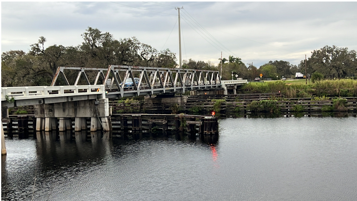
Figure 4.47: Fort Denaud Swing Bridge showing no sign of damage. Coordinates: 26.74411, -81.51015
