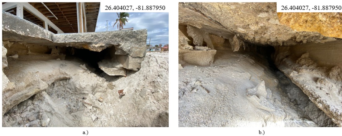
Figure 4.35: Ground photos of failures observed in south east end of the Fort Myers Beach island, at Carlos Point Condominium Associates: (a) ground photos of the erosion beneath the foundation depicting the scope of eroded area; (b) ground photo of the underneath the foundation depicting the exposed footing
