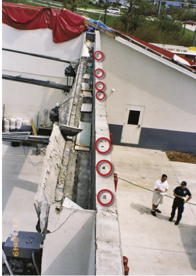
Figure 2.9: At Fire Station No. 12, the tie-beam storm anchor straps for the roof truss failed in Port Charlotte. Coordinates: 27.00927, -82.035509. (Ingargiola et al. , 2005)
