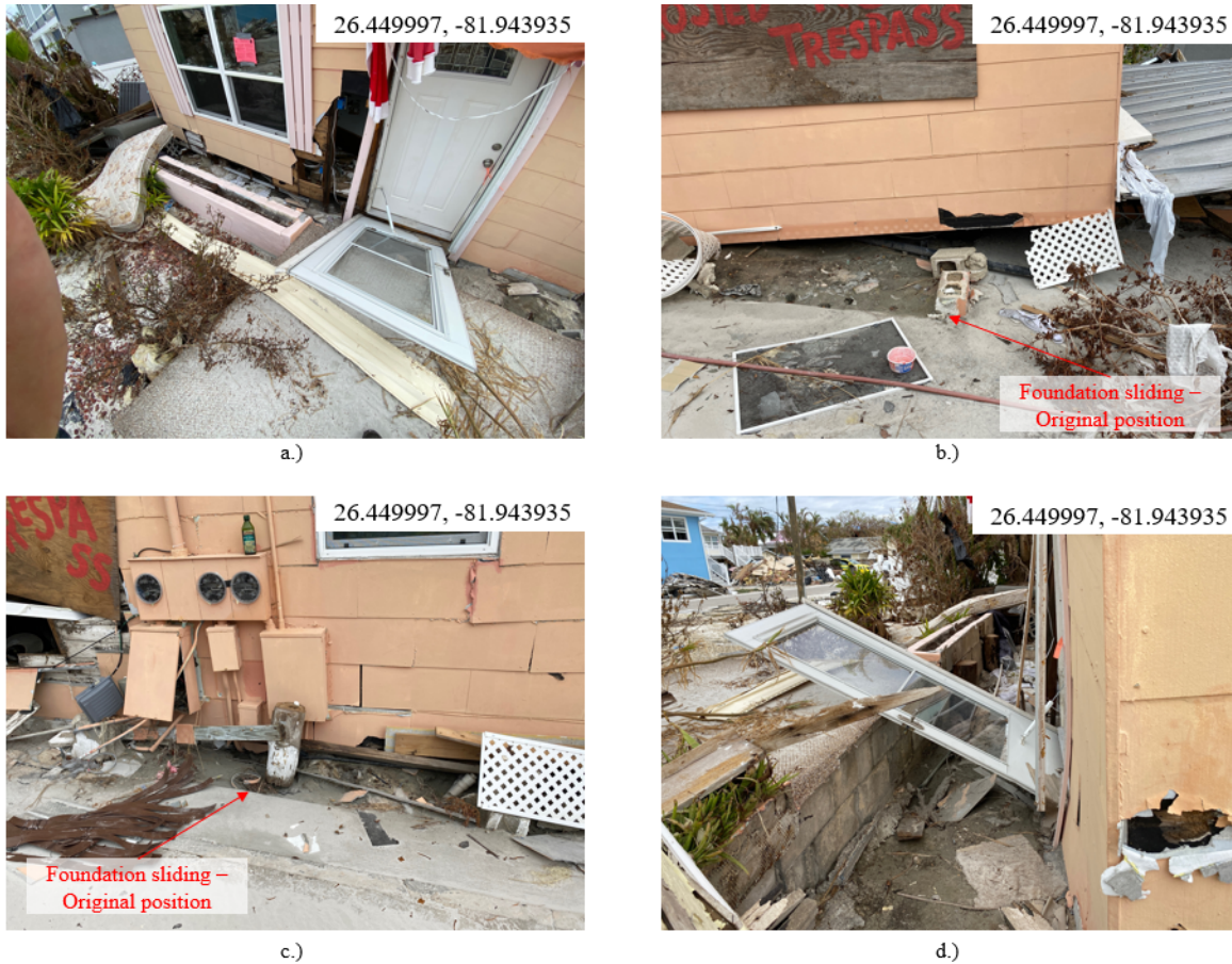
Figure 4.42: Ground photos of the failures adjacent to Estero Blvd in Fort Myers Beach: (a) front of the residential building showing that foundation has slid; (b) right side of the residential building showing that foundation has slid; (c) right side of the residential building showing that foundation has slid; (d) left side of the residential building showing that foundation has slid
