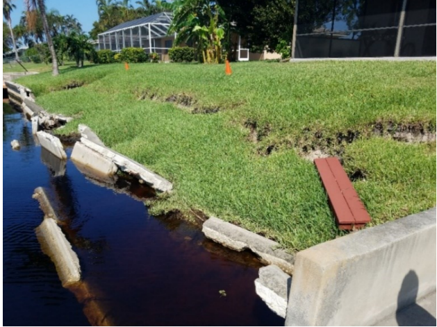
Figure 2.13: Seawall collapse at Cornwallis Parkway in Cape Coral. Coordinates: 26.595572, -81.930611 (Stark & Hudyma, 2017)
