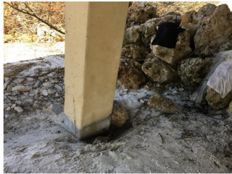
Figure 2.16: Bridge scour at the base of the piers, Big Carlos Pass Bridge. Coordinates: 26.404081, -81.878197 (Stark & Hudyma, 2017)
