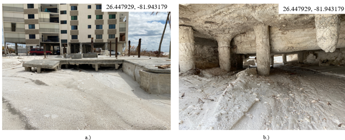
Figure 4.40: Ground photos of failures observed in north west end of the Fort Myers Beach island near Pelican Watch Condominium: (a) scour and erosion under the shallow foundation of a building; (b) Close up photo of damage to shallow foundation
