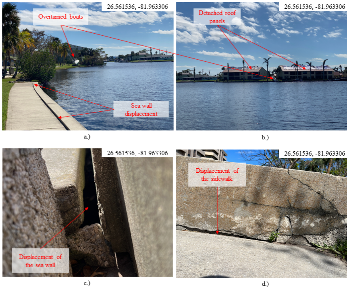
Figure 4.21: Ground images of Four Freedoms Park: (a) Overturned boats as a result of extreme water surges and wind power along with slight displacement of the sea wall along the side walk; (b) due to Hurricane Ian's powerful winds, roof panels came off as evidence of a structural failure; (c) closer look at the displacement of the sea wall; (d) the displacement also came from the base where there were stairs.
