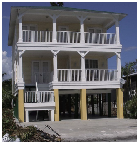
Figure 2.7: No storm surge damage was done to a newly built house perched on piles in Fort Myers Beach. Coordinates: 26.97066, -82.08998. (Ingargiola et al. , 2005)
