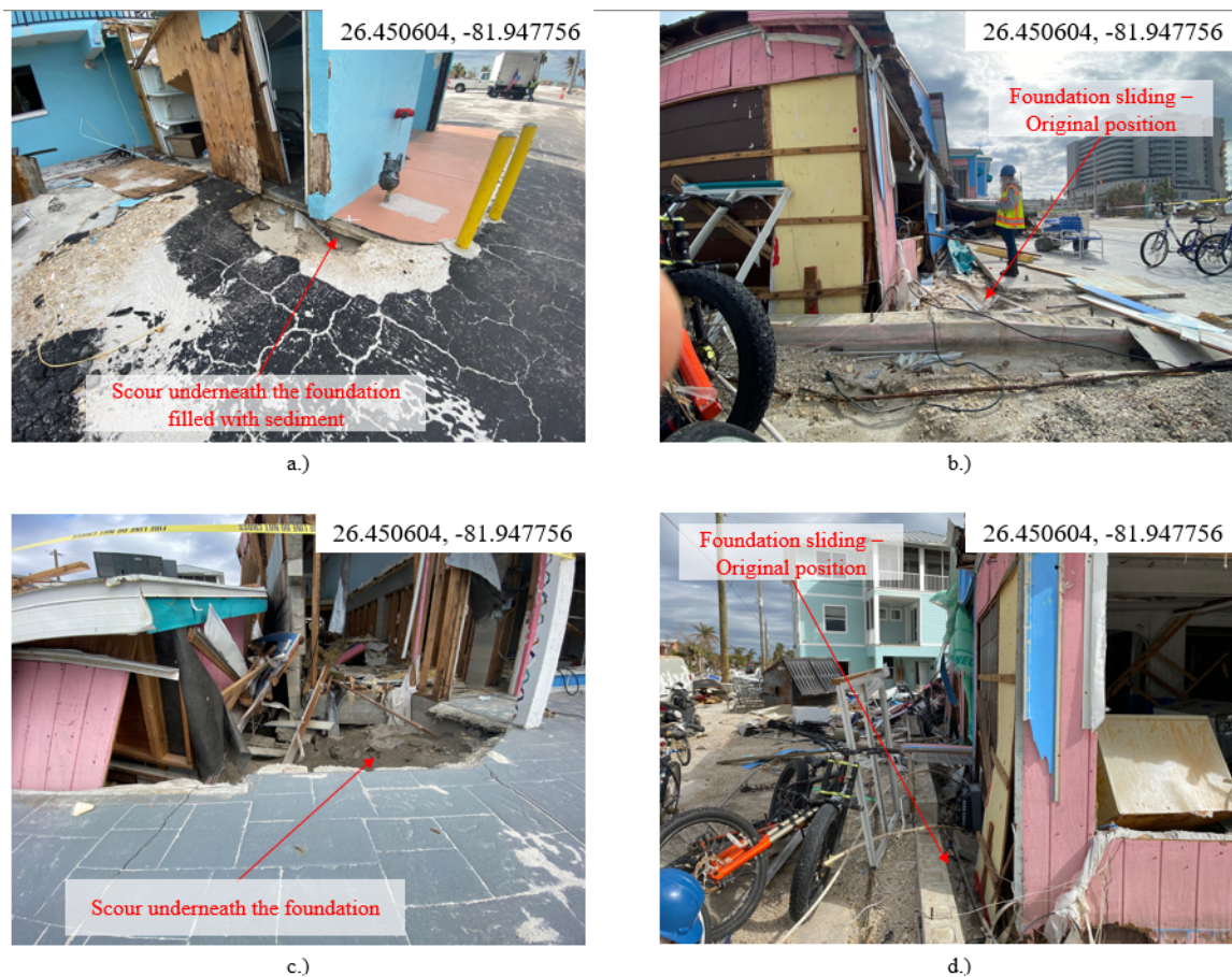
Figure 4.41: Ground photos of the failures adjacent to Estero Blvd in Fort Myers Beach: (a) photo of a shop building depicting erosion beneath the foundation; (b) sliding of the front of the building as a result of the scour and erosion behind the building, beneath the foundation; (c) scour underneath the foundation at the back of the building causing a cavity and engulfing the back of the building; (d) image showing the left side of the building sliding
