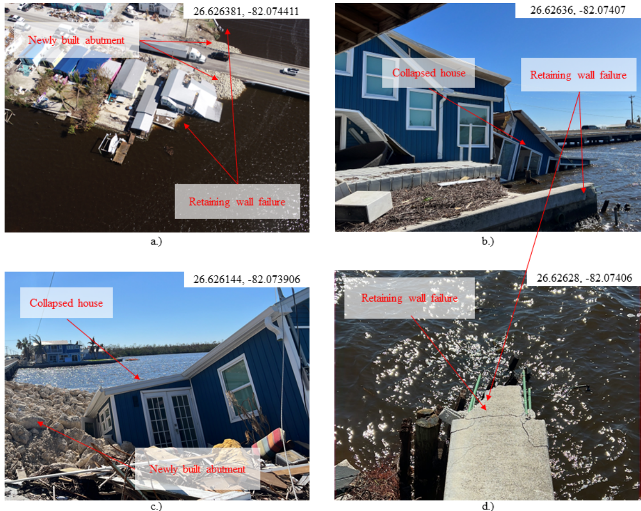
Figure 4.11: West entrance to Matlacha: a.) drone image of a severe retaining wall failure on both sides of the bridge along with the newly built abutment; b.) ground photo of the back of the house showing the remaining section of the retaining wall and the magnitude of collapse caused by the failure leading to half of the house sinking; c.) ground photo showing the road front of the house with the abutment built after the collapse; d.) Plan ground photo of where the retaining wall failed behind the house.
